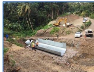
Despite these challenges a number of tasks were accomplished at the end reporting quarter. This includes (i) completion of the assembly of the bridge, (ii) backfilling of the bridge, (iii) 90% completion of the retaining walls and (iv) 50% completion of the drainage system. Despite the challenge of being six weeks behind the planned schedule, the project is deemed 70% completed at the end of this reporting period, with expenditure standing at EC\$0.88M.
