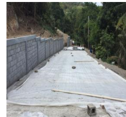
Figure 1: Concrete Road Retaining Wall Construction
