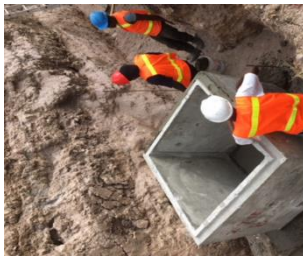
Figure 3: Installation of pre-cast manholes
