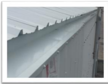
Figure 4: New Roof Sheeting and guttering system
