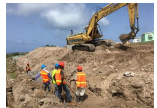
Figure 2: Excavation of trench
